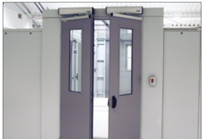
Double wing doors with automatic door handle
