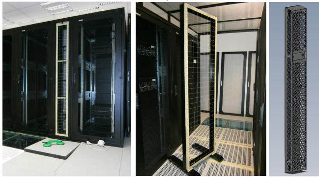
The measurement at the air intake of the cooling unit has shown that the change of air-flow will not be significant. The more narrow rim on the front door frame is not so big change to see dramatically increased air-flow.
